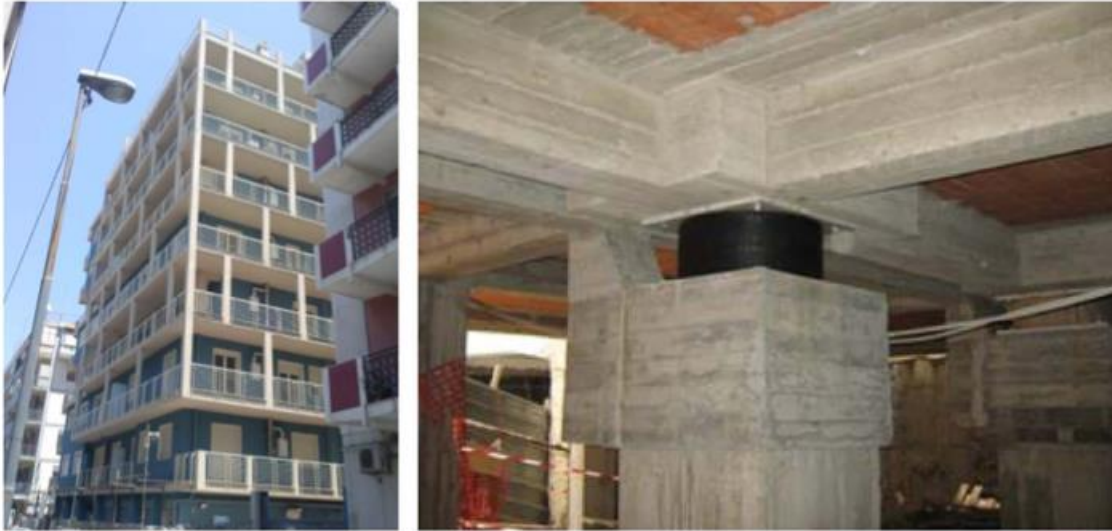
Figure 9. The residential building in Spatafora Street in Messina, which is the tallest seismic isolated building in Italy.
