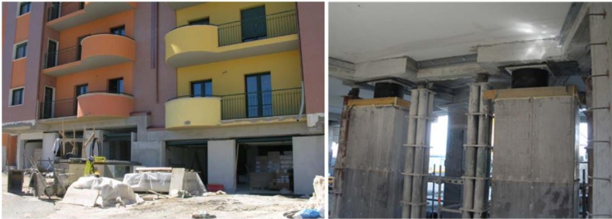
Figure 17. The reinforced concrete buildings in Pianola, L'Aquila (courtesy of FIP Industriale)
