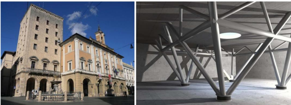
Figure 22. TMD at the top of the Civic Tower in Rieti
