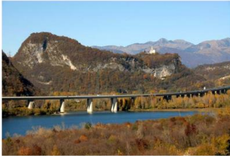
Figure 3. The seismically isolated Sompago viaduct of the Udine-Tarvisio freeway, after its completion, Italy.
