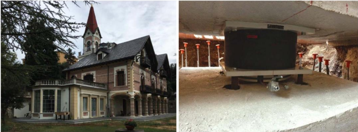
Figure 20. View of the historical masonry building called “La Silvestrella”, L’Aquila, and a HDRB
