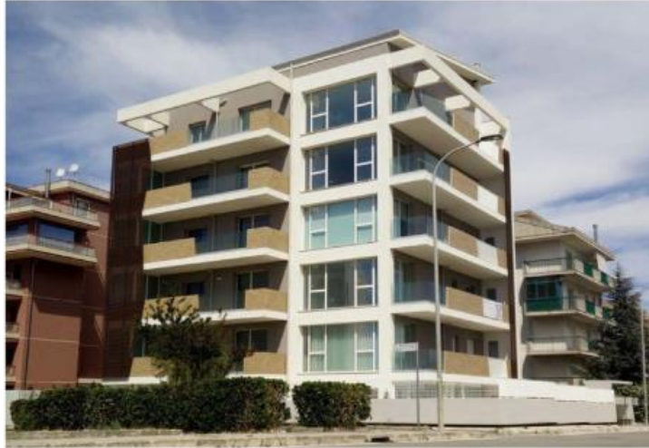
Figure 10. The “120 Forlanini” residential building in Ragusa (Courtesy of FIP Industriale)
