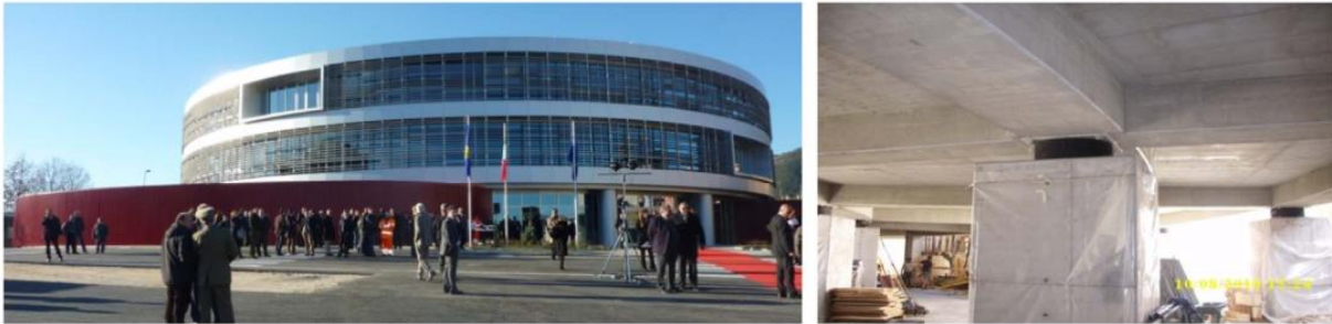
Figure 7. The ANAS building in L'Aquila
