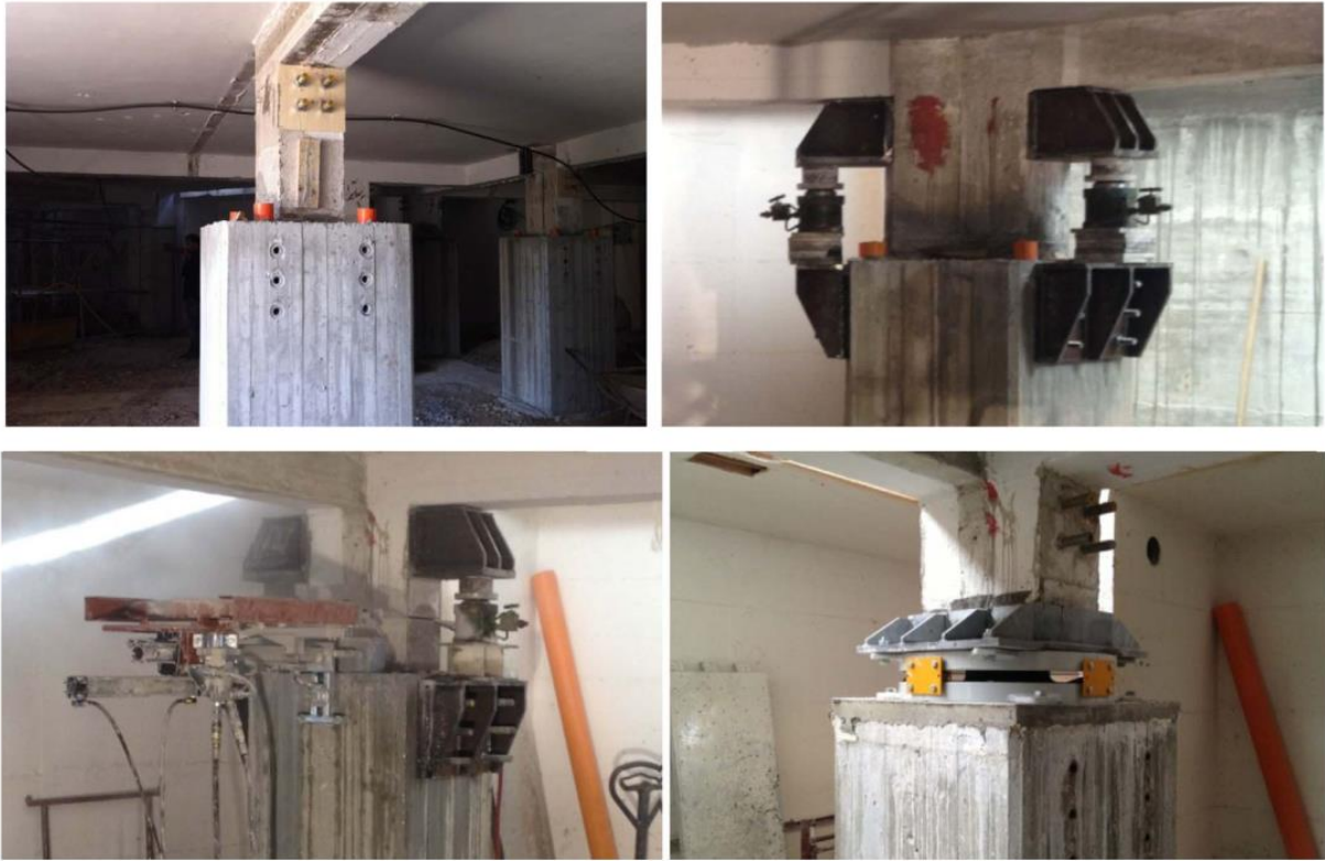
Figure 16. Leonardo building. Insertion of an isolation device (courtesy of FIP Industriale).
