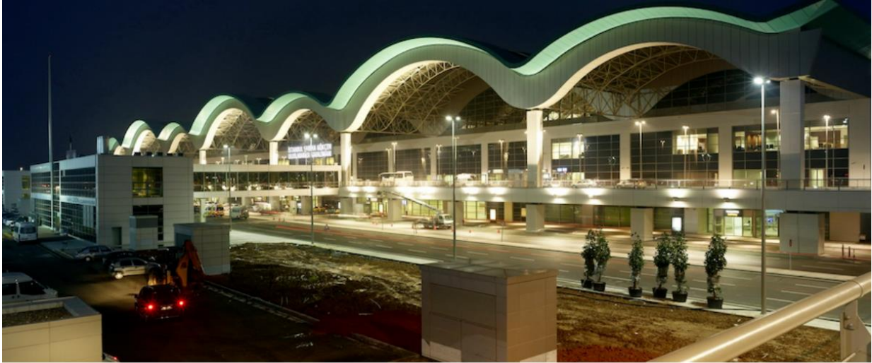
Figure 43. Sabiha Gökçen Airport International Terminal, Istanbul
