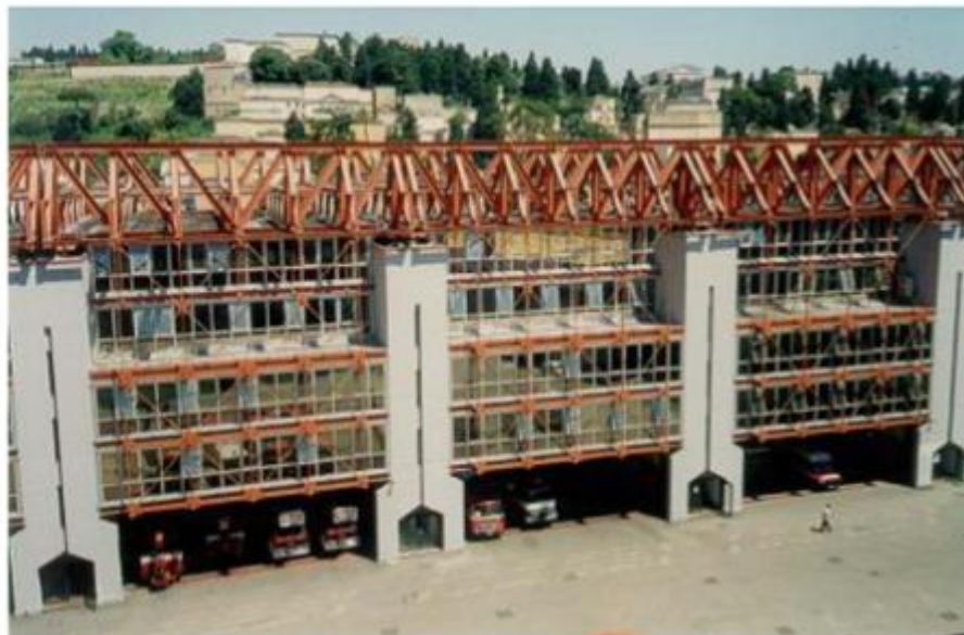
Figure 4. The first seismically isolated fire-command building in Naples, Italy
