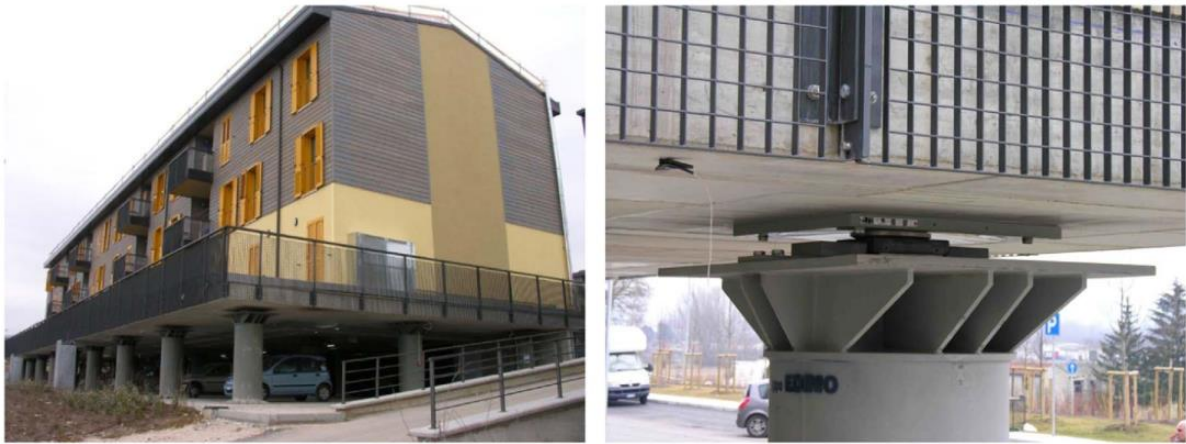
Figure 6. One of the buildings of the C.A.S.E. project, isolated by means of Italian CSSs in 2009
